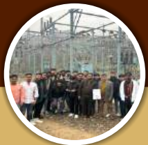
Industrial Visit to HVDC Terminal Station, Padghe
